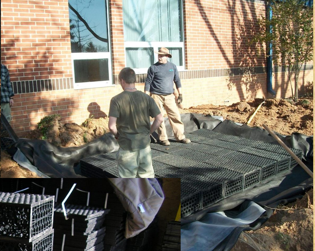
Installation of Bio Boxes
